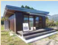
南GO!! Station (庁舎西側)
